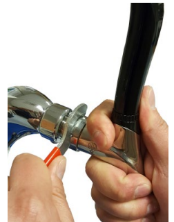
Tighten shank nut with faucet wrench
