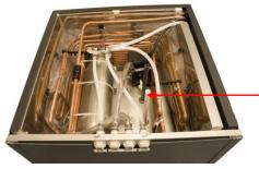
Water level should be 1/4" below white overflow pipe stem
