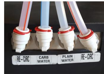
**Step 5:** If you are comfortable your connections are leak-free, wrap the exposed hoses and fittings with the insulated tape and push the unit in place.
