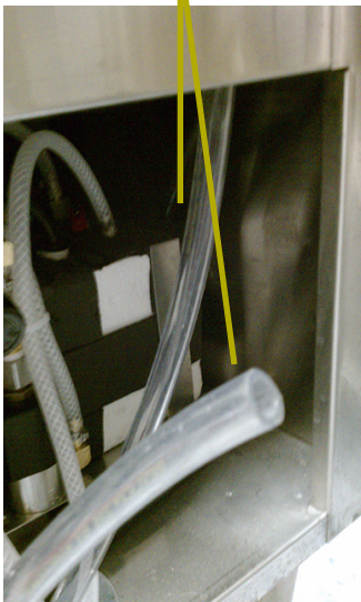
3/8" Drip pan drain hose. Located out the back of the unit. 6' length.
