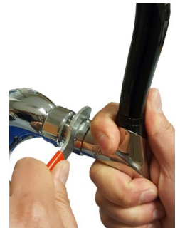
Tighten shank nut with faucet wrench
